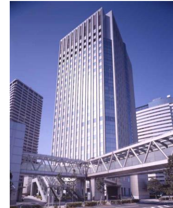
Office Building 25.331 m 2 Tenant-Occupied
